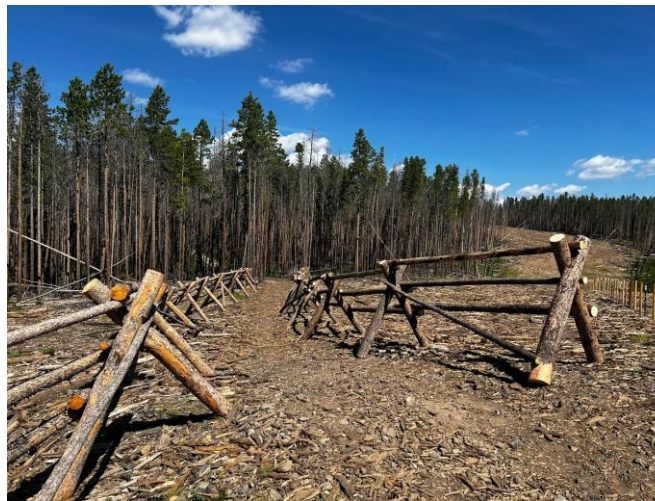
Buck and rail fence along UTV trail
